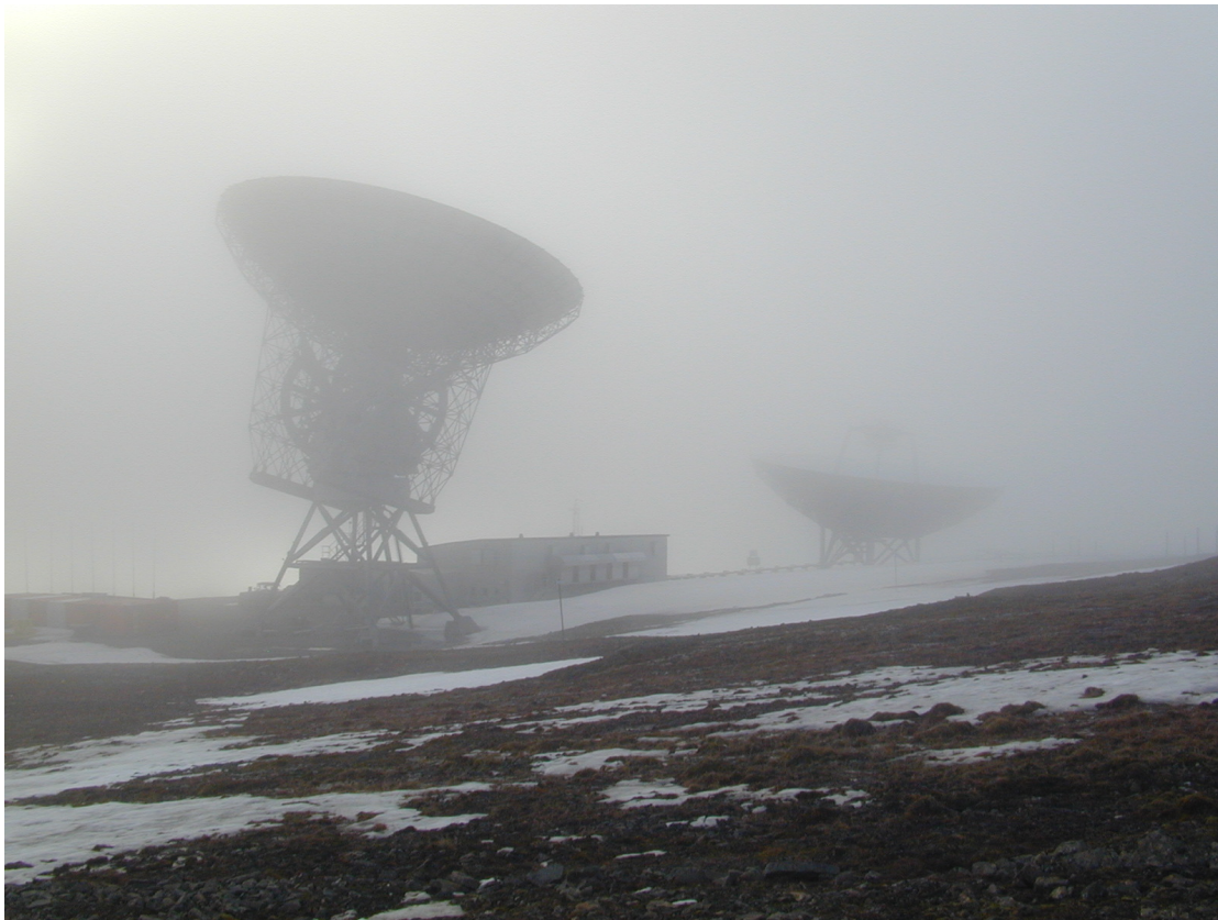
Figure 31: STEFFELEO: ESR antennas , in the early hours of July 9, 2006. The 32 antenna (left) is pointed towards East, azimuth 90^\circ , at 75^\circ elevation. The magnetic-field-aligned ESR 42 m antenna (right) was not used in the beam park measurement.
